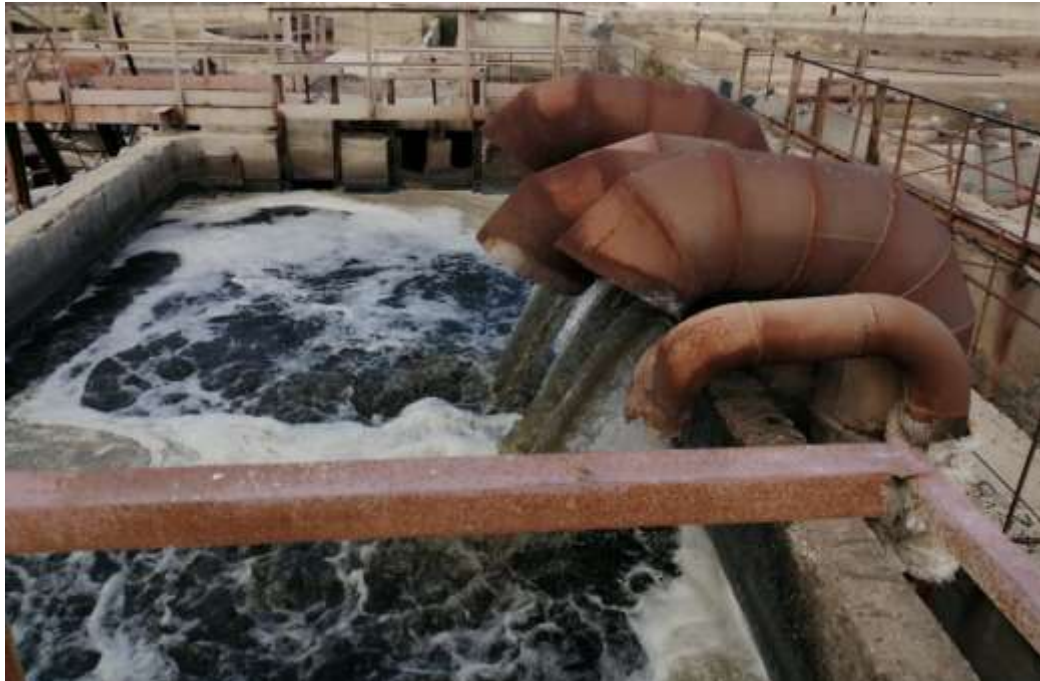
Fig. 2 - STP -1 aeration tank
