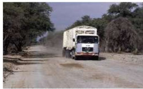
Road reshaping is required to restore camber
